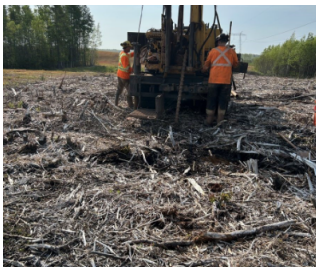
DRILLING WITHIN CLEARED ROW
