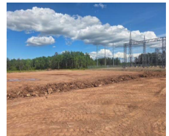
EXCAVATIONS TO SUBGRADE AT MEMRAMCOOK
